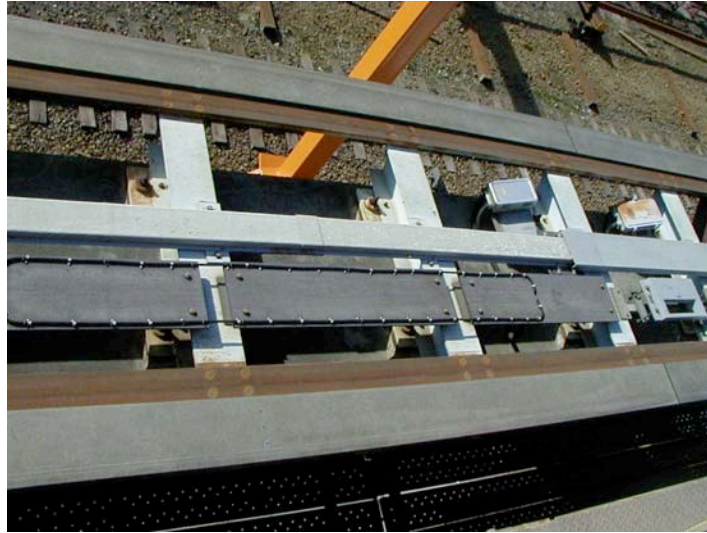
Figure 3-2. Overall View of Guideway at Test Track
