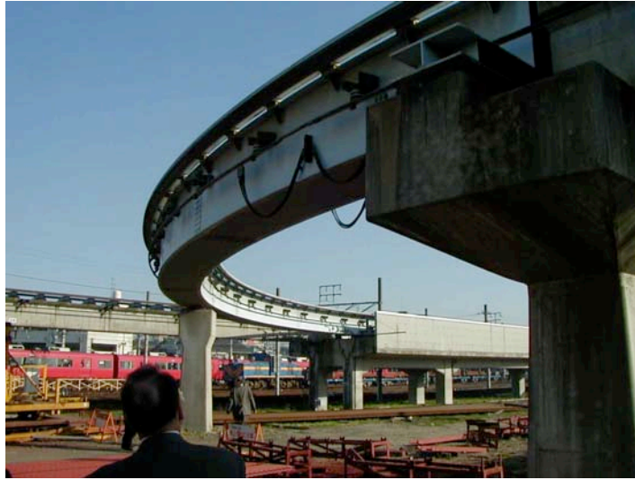
Figure 3-11. 25 m Radius Curved Guideway Leading Into Switch
