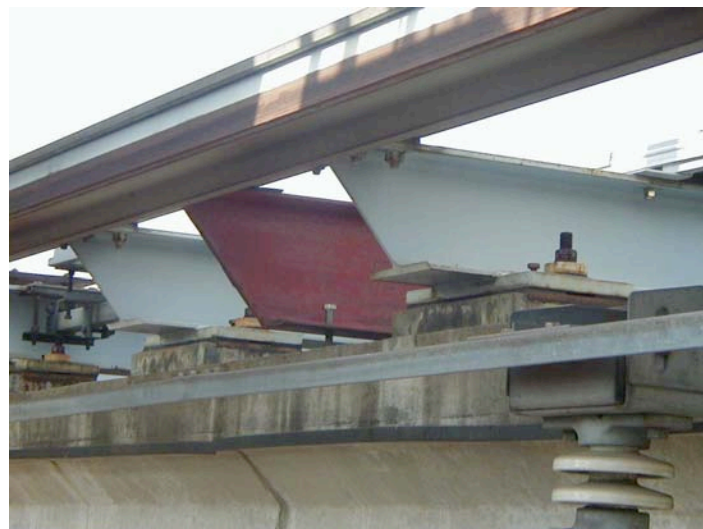
Figure 3-3. Guideway Rail and Sleeper Supports
