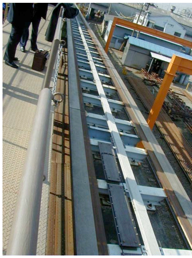
Figure 3-5. Sleeper Spacing for Guideway Rails
