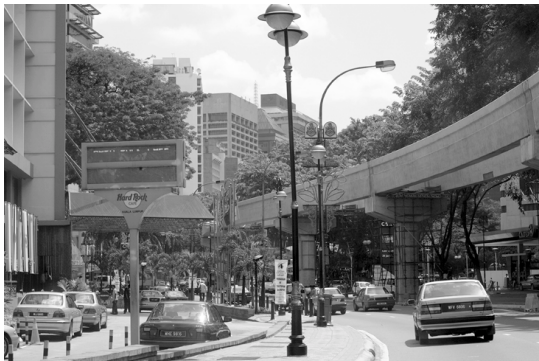
Monorail guideway in Kuala Lumpur, Malaysia.
