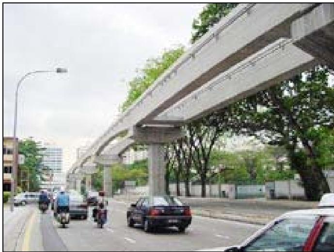
Figure 2.4—Kuala Lumpur monorail guideway has both straight (foreground) and arched (background) segments.
