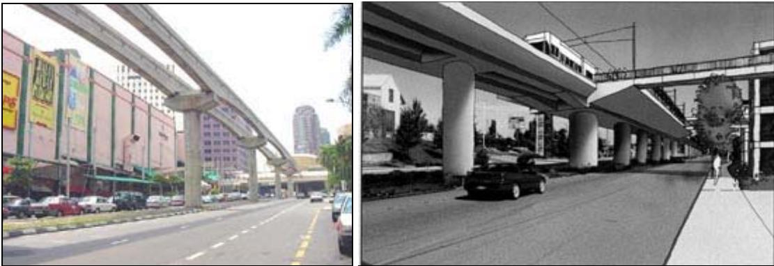
Figure 3.6—Monorail has the lowest impact of any elevated rail system. Notice the difference in shadowing effects between monorail and light rail aerials (Kuala Lumpur guideway (right), Projected Seattle light rail aerial (left)). Source: Monorail Malaysia/ Sound Transit.
